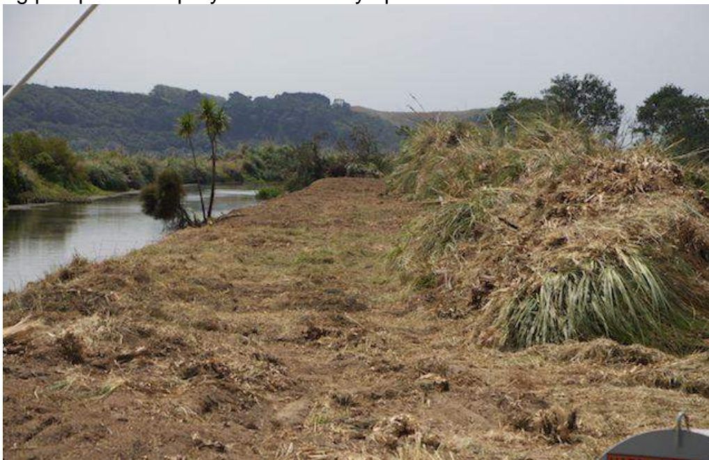
First day of operations - Wharere Canal stopbank.
